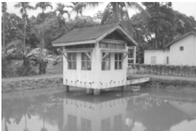
Fig. 2. A concrete house for poultry cum fish culture
